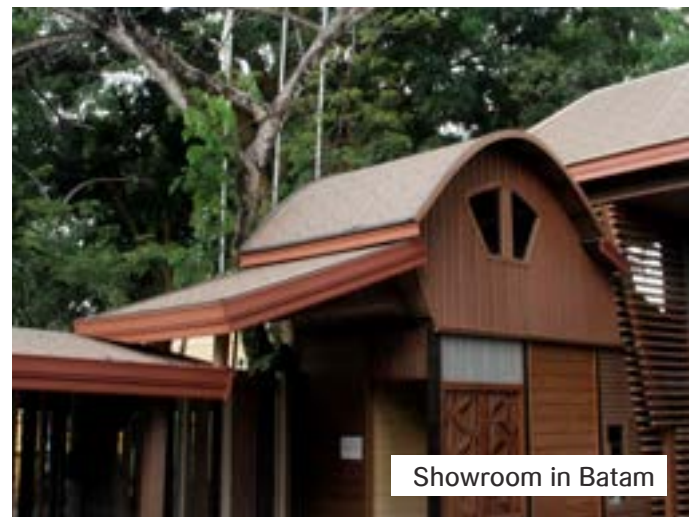
Showroom in Batam
